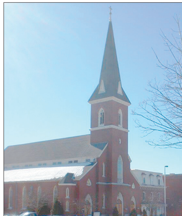
St. Joseph's Church and rectory on Main Street in Lewiston in 2011. The Church on the National Register of Historic Places has a reprieve from demolition; the rectory does not. (Photo by Rachel Morin)
