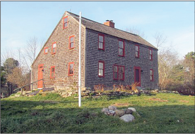
One of Freeport's oldest structures, the Greenfield Pote House was built in Falmouth c.1760 and moved to its current location by boat in 1787. (Photo courtesy of Wolfe's Neck Farm)
