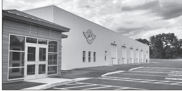
Hartt's new 30,000-square foot facility in Kitty Hawk Business Park boasts state-of-the-art features.
