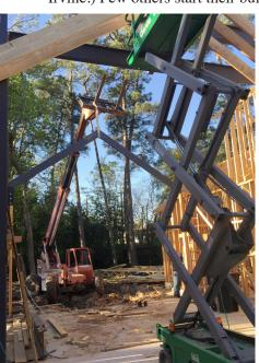
a large custom home when the contracted builder disappears. And few others have designed and patented a construction process using prefabricated metal framing to be able to construct extraordinarily large and affordable luxury homes.
