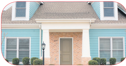
222 James Longstreet Blvd. - Looking for all the amenities with none of the outside work? This beautiful town home is perfect for anyone who doesn't have time to maintain an exterior appearance but needs the space. 2 car garage*open floor plan*loft/walk-in closets up/ downstairs*pantry. MLS#1807060 $158,900
