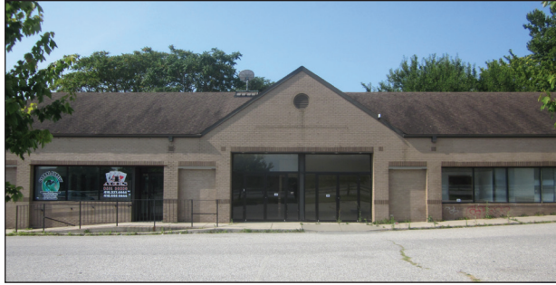
Charm City Medicus LLC is currently renovating this building on North Point Boulevard for a marijuana dispensary.
