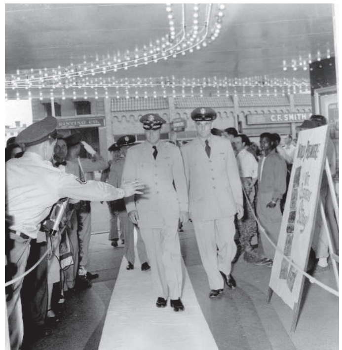
PHOTO COURTESY OF SELFRIDGE AIR NATIONAL GUARD BASE
