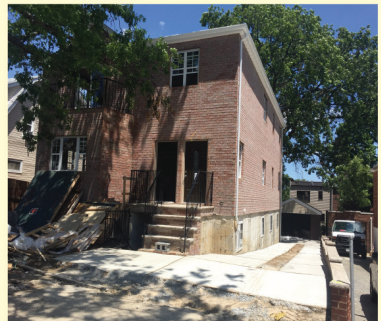
THROGGS NECK BRAND NEW LUXURY 2 FAMILY BRICK WITH FINISHED BSMT 4500 SF OF LIVING SPACE 2 THREE BDRS 2 BATHS APTS W/ LAUNDRY & PORCH FINISHED BSMT W/ FULL BATH & PRIVATE ENTRY GARAGE $975,000
