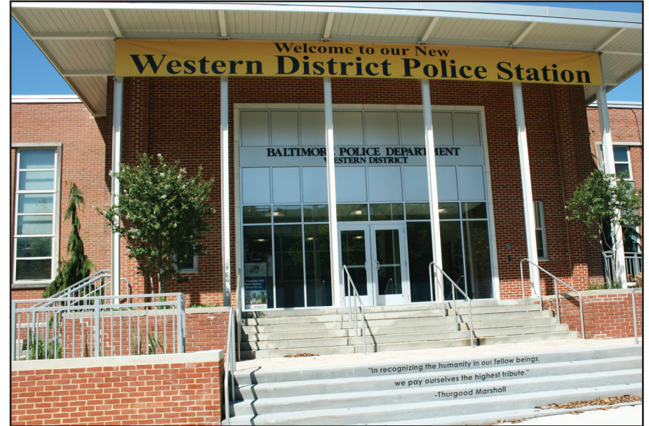
Newly renovated Western District Police Station Photo: Dennis Roberts
