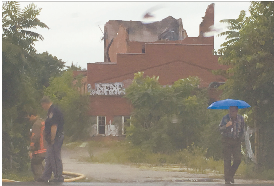
Firefighters and police officers remained on the scene of a still-smoldering building at the former Seagram's property Tuesday morning.
