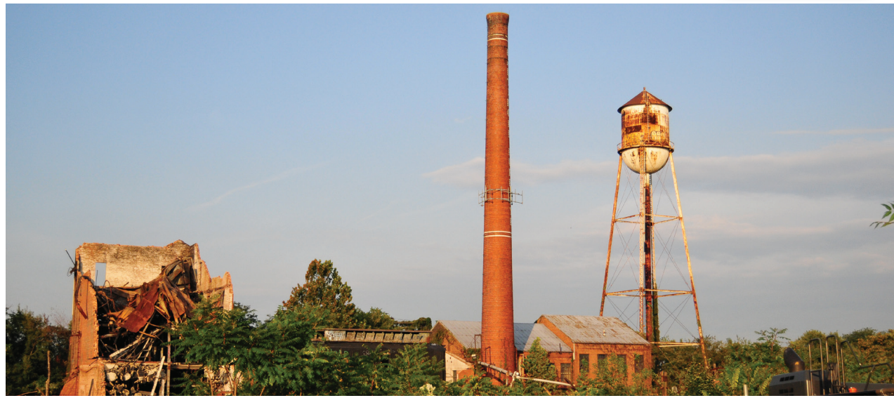
As of Tuesday morning, Sept. 5, all that could be seen still standing on the property was one intact building between the smokestack and water tower and the remnants of another that had been partially demolished. The smokestack and water tower are historically designated and will remain standing on the property. Photo by Marge Neal.
