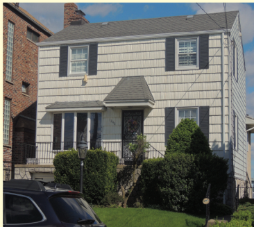
LOCUST POINT WATERFRONT COLONIAL CHARMING 3 BDRS 2 BATHS W/ FAMILY ROOM FIREPLACE PORCH PATIO DOCK 350 FT REPAIRIAN RIGHTS PANORAMIC VIEWS THE TN BRIDGE $849,999
