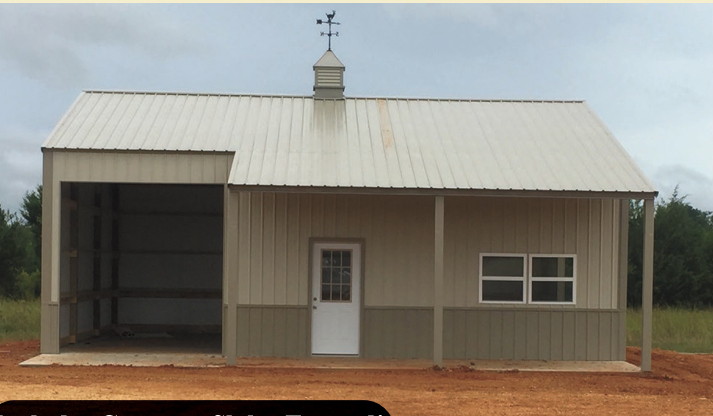
Includes Concrete Slab - Erected!
