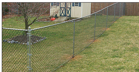
Chain Link Fence
