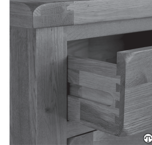
Traditional dovetail joints provide tensile strength at the drawer front.
