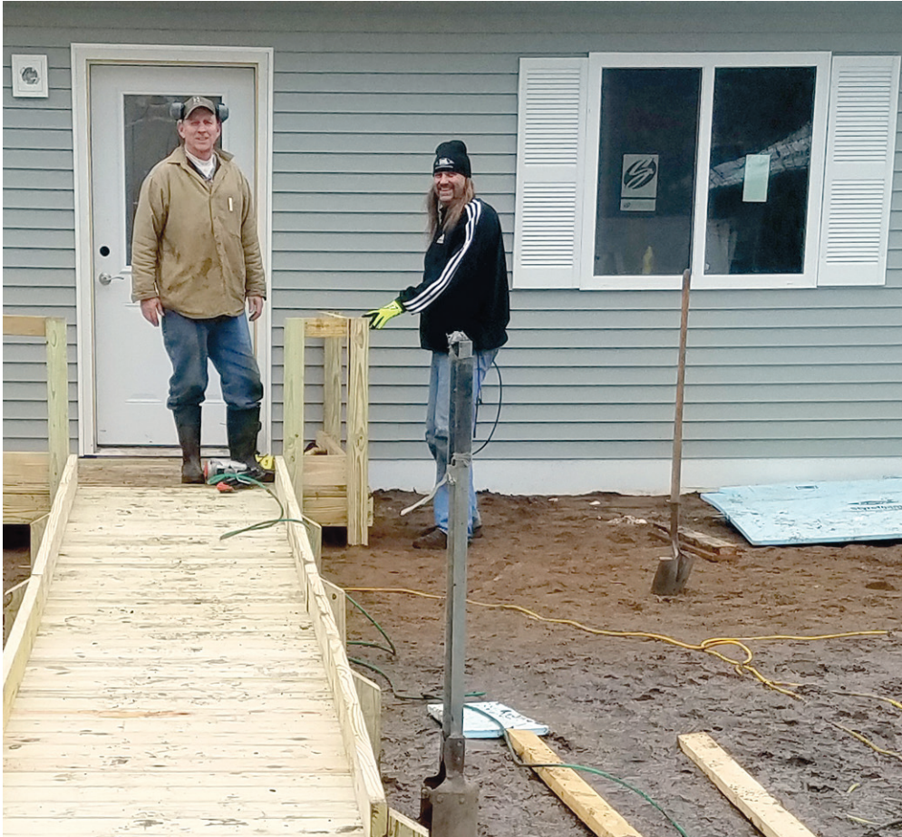
Tim McCarthy, LAIC construction manager and a volunteer rush to complete a wooden 12-foot ramp on the back deck and (here) ramp on the front deck with a 40-foot wooden sidewalk for the wheelchair-bound homeowner.
