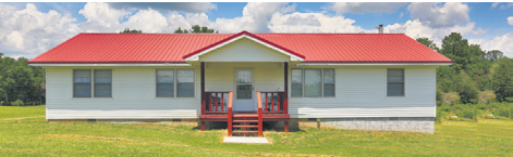
T-1353: 34383 Ardmore Ridge Rd, Ardmore. Nicely remodeled home situated on 17.7 acres, 1798 SF, 4 BR/2.5 BA, laminate & tile flooring, crown molding & updated covered back porch + above ground pool. 40x60 metal shop and fencing for horses. MLS#1848539 $229,900.
