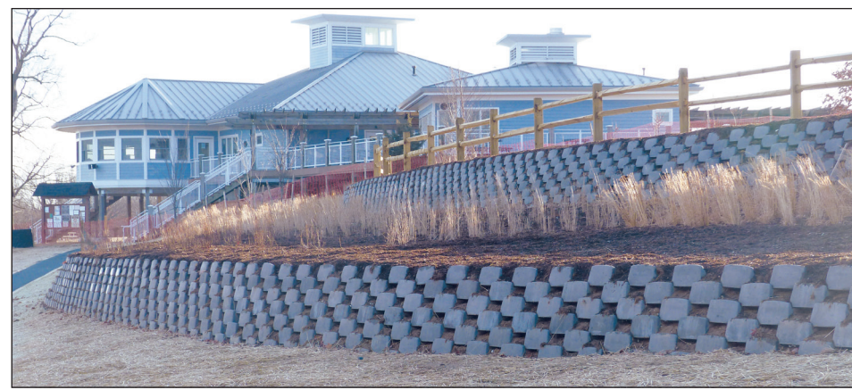
Due to the design of the blocks, all of the spaces within the wall can be seeded with plants to grow in and actually make it stronger. And a new path directs visitors around the wall.
