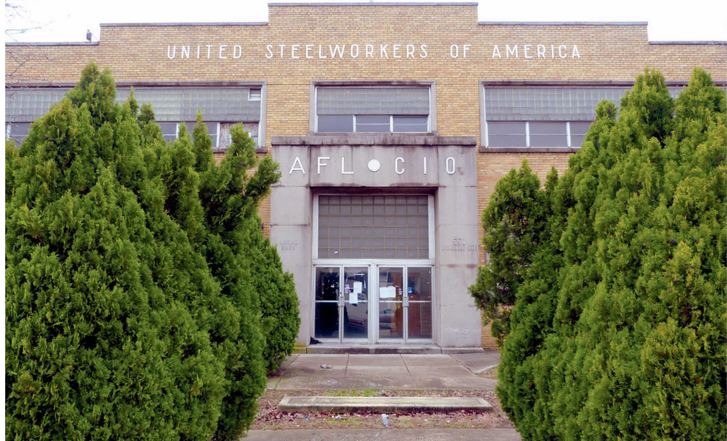
Following the sale of the former steelworkers union building at 550 Dundalk Ave., the operators of a food distribution program for the needy have not been allowed back inside by the new owner to retrieve their property. Photo by Devin Crum.
