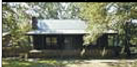
610 COUNTY ROAD 241, MOULTON
