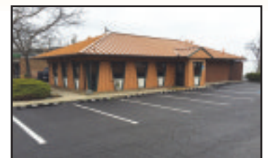
Sheffield Lake 4175 E Lake Rd. 1740 SF retail building w/Lake Erie views!
