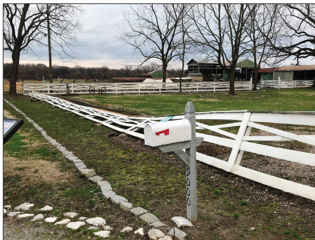
Left: Much of the wooden fence had fallen down following heavy winds on March 2, but volunteers determined the fence posts were likely rotted below the ground. Right: After weeks of planning and repairs, the fence is back to its former glory. Courtesy photos.
