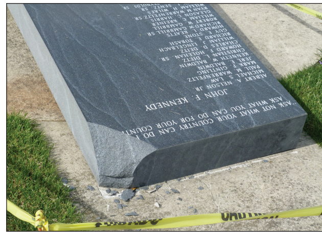
A top corner of the slab broke off on impact, meaning the monument could not be repaired.
