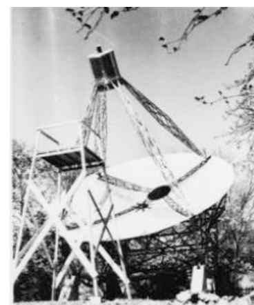
Grote Reber's Radio Telescope 1937
