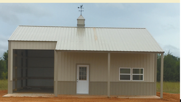
Includes Concrete Slab - Erected!
