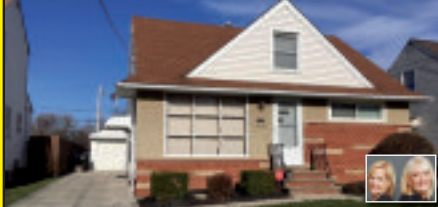
17809 Crestland Rd. CLE Newer windows & concrete Drive $89,900
