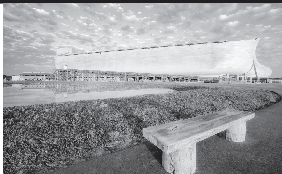
The Ark, the largest timber-frame building in the world, is made up of three decks that include teaching exhibits and displays of incredible craftsmanship.
