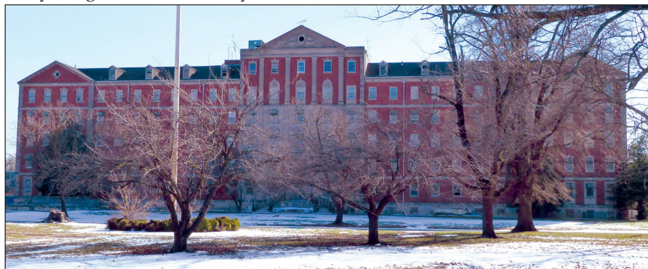
Now dilapidated, the entire main structure of the hospital building will have to be restored for historic preservation. File photo.
