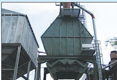
Refurbished 30 Unit Bin
