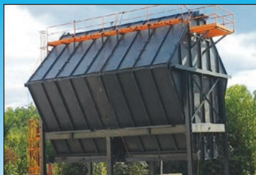
Refurbished 62 Unit Bin
