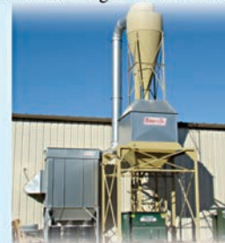
Round and Square Pulse Jet Baghouse Filters from 1,000 to 61,000 CFM
