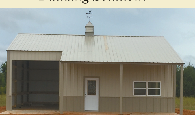
Includes Concrete Slab - Erected!
