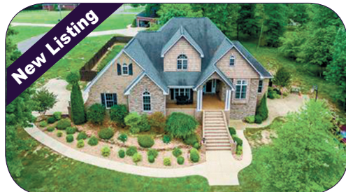
New Listing 61 Windwood Dr. - EXPERIENCE THIS IMMACULATE CUSTOM BUILT HOME in Windwood Subd! Unique features throughout & excellent construction. WOW when you walk in to the Great room w/fireplace, HUGE master suite, granite countertops, & fin basement w/office/bedroom, walkin closet, full bath/rec room & extra garage area. Large Second story bedrooms w/jack n jill bath. MLS# 1929265 $385,000
