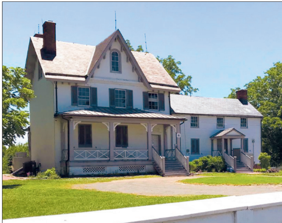
A total of 12 panes were replaced in the Todd house's second-story windows before being professionally reglazed. Courtesy photo.
